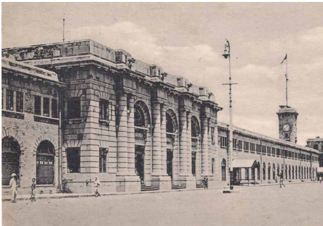
Mole Station at Ballard Pier was built by the Bombay Port Trust in the neoclassical style with Doric columns and classical ornamentation on the entablature
